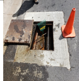
Inside of north SD Box. Stagnant, stinky, murky water was scooped out and also drained. No visible inlets or outlets.
