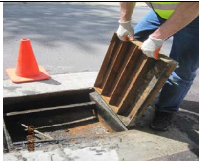
Inside the South SD box- found completely dry and empty. Ribbed steel lid. Possible proposed catch basin for Willow Lane.
