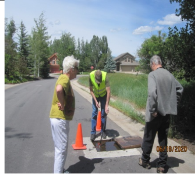
Inside North SD Box – found it full of murky, immiscible street water. 30" from ground to plywood divider; 14" from plywood to road. Total 44".
