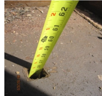
South SD box , 56" from ground to plywood divider + 12" up to road, total 68". No inlets or outlets.
