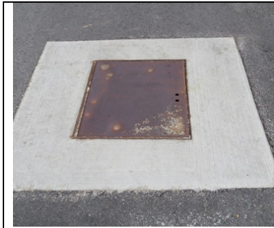
SOUTH SD box near SS Lot 138 SW Corner on Ranch Place (road) and Willow Lane. Square steel lid.
