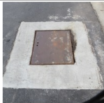
NORTH SD Box – 130' north from South SD Box. In front of Lot 154. May be catch basins for this road.
