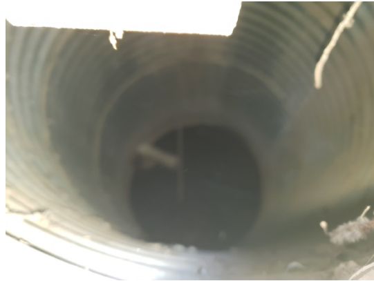
Exterior uncovered lip of drain and cover. Interior photo taken with camera probe. Found to be Dry.
