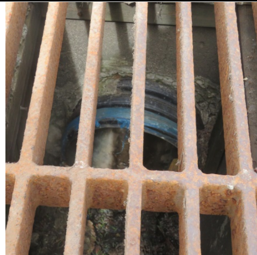
Storm Drain grate SW corner 23.5 feet.
