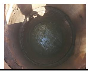
**Mh 17A** Located at Lot 48, Groth. Lake Front Court. Steel lid exposed at grade. West side of driveway, near curb, next to large flat boulders. Lid has a metal ring on the top center. Rarely inspected. **Inactive**.
