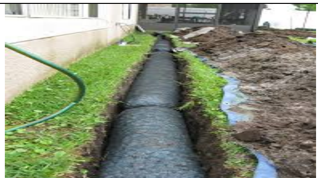
Figure 3 Adding French drains years after construction
