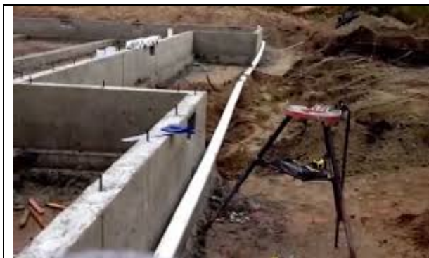
Figure 2 Beginning construction- concrete forms alongside of French under drain pipes.
