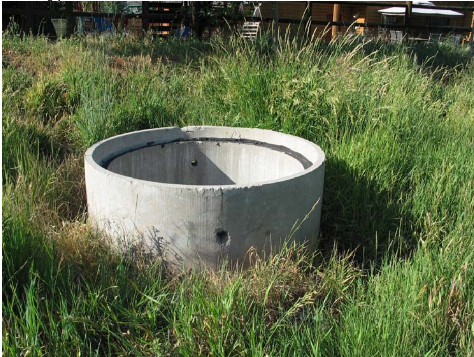
Parcel J culvert . View from outside
