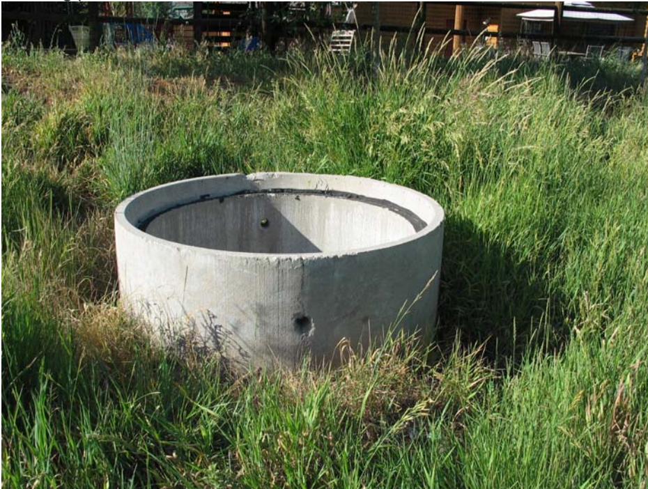
Parcel J culvert . View from outside
